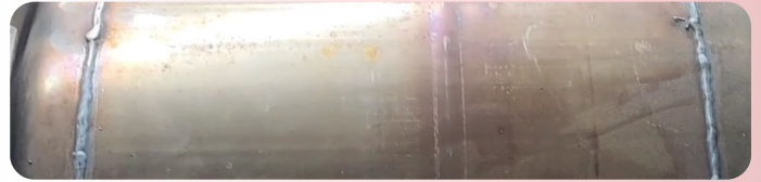
SCR substrates replaced, but no indication of Type Approval or Homologation number.
